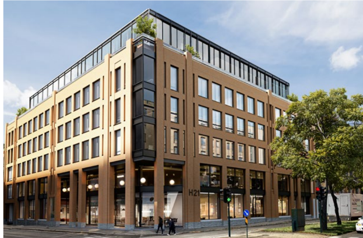
Hausmanns gate 21, Oslo 10 836 m 2
